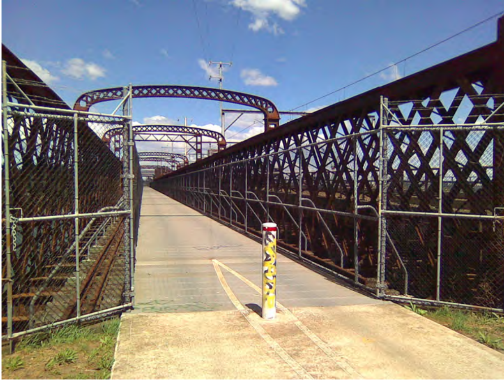
John Whitton Bridge Cycleway Meadowbank, Sydney
